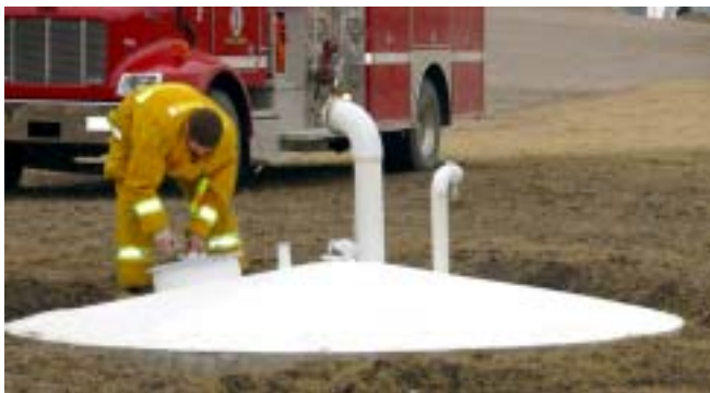
Figure 2. Storage tanks are located close to roadways and vary in type — some horizontal and completely buried, and some vertical tanks with their tops exposed. Most of the tanks were acquired for little or no cost to the fire department.
